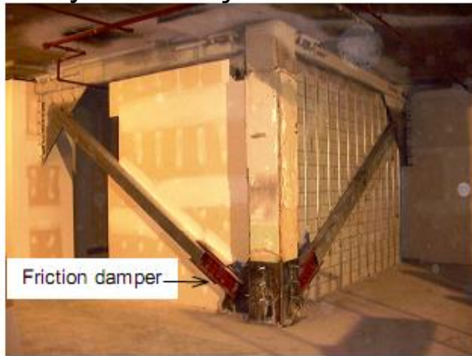
Figure 4. Friction damper in single diagonal brace.
