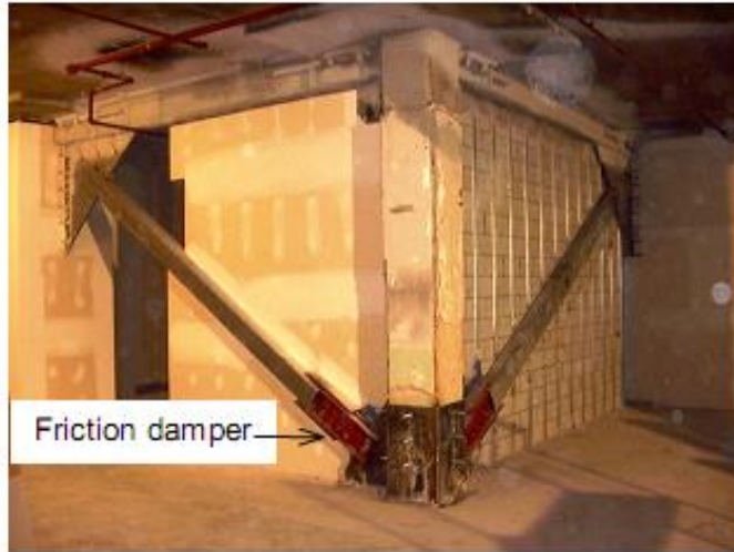
Figure 4. Friction damper in single diagonal brace.
