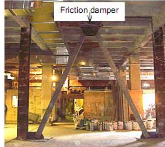
Figure 5. Friction damper at top of chevron brace.
