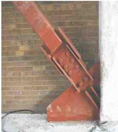
Friction damper in single diagonal bracing
