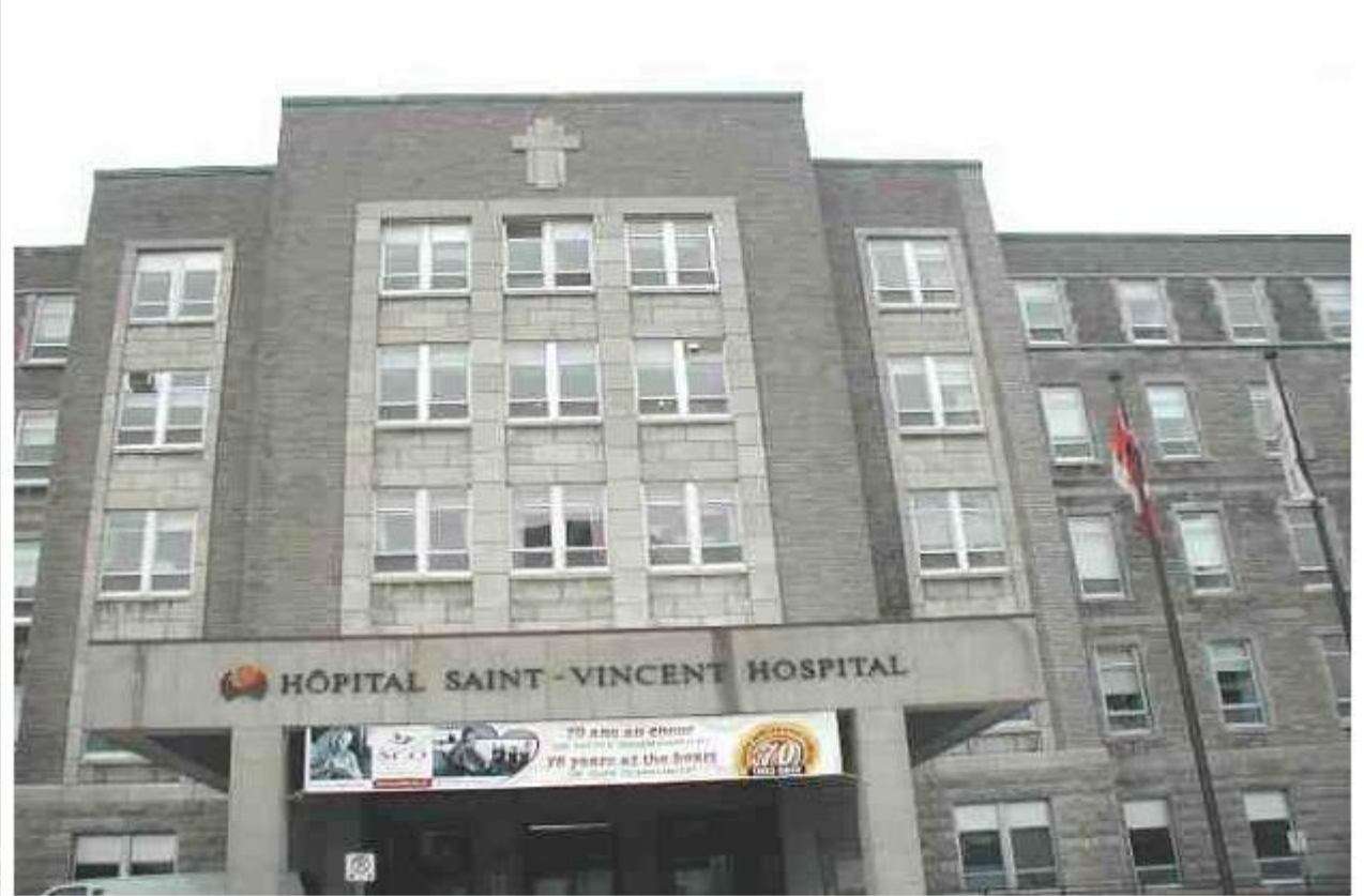
Figure 1, Front View of Wing-B (Partial)
