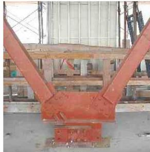
Friction damper in chevron bracing (inverted)
