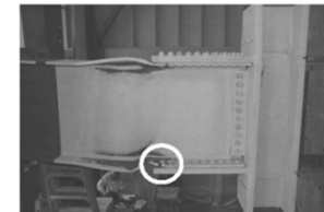
(a) Fracture Location
