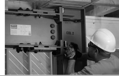
Fig. 12.1. Simpson Strong-Tie Strong Frame moment connection.
