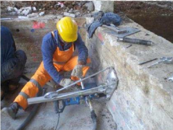
CONNECTION BAR DRILLING
