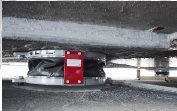
INSERTION OF SEISMIC ISOLATORS
