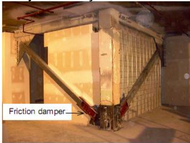
Figure 4. Friction damper in single diagonal brace.
