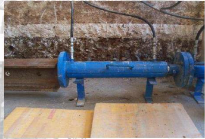
STEEL BEAMS DRIVING
