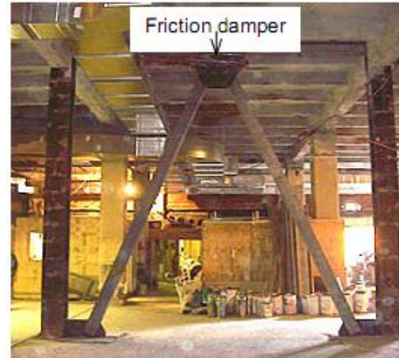
Figure 5. Friction damper at top of chevron brace.
