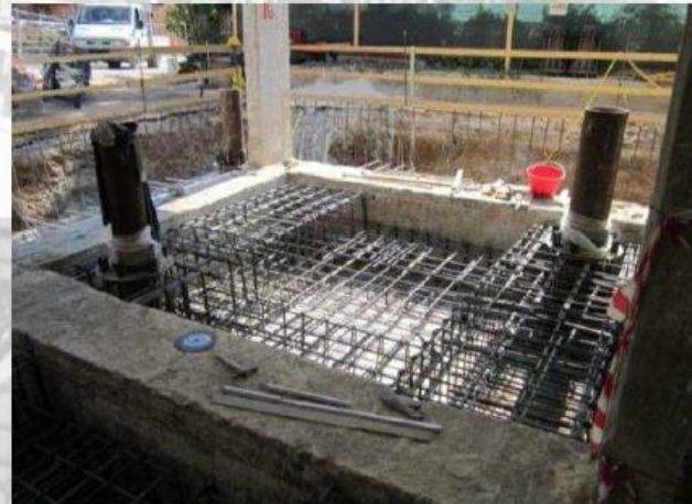
UPPER SLAB REINFORCEMENT and
