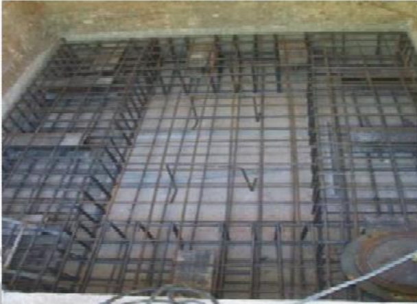
BOTTOM SLAB REINFORCEMENT
