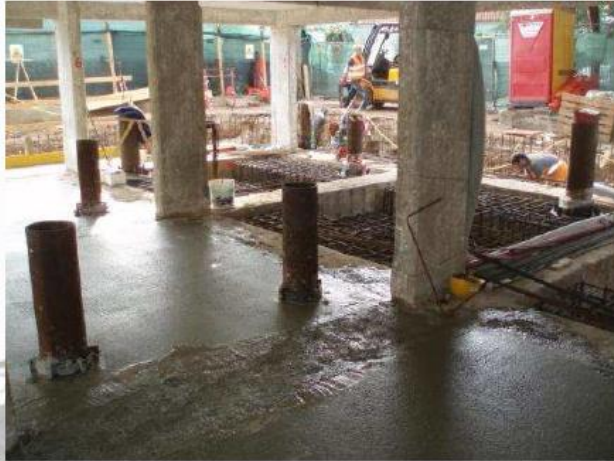
CASTING OF UPPER SLAB
