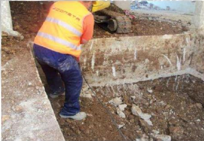
REMOVAL OF EXISTING FLOOR
