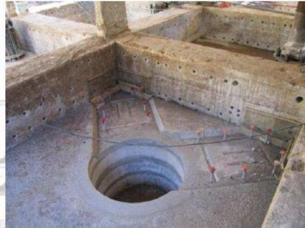
MANHOLES IN THE BOTTOM SLAB
