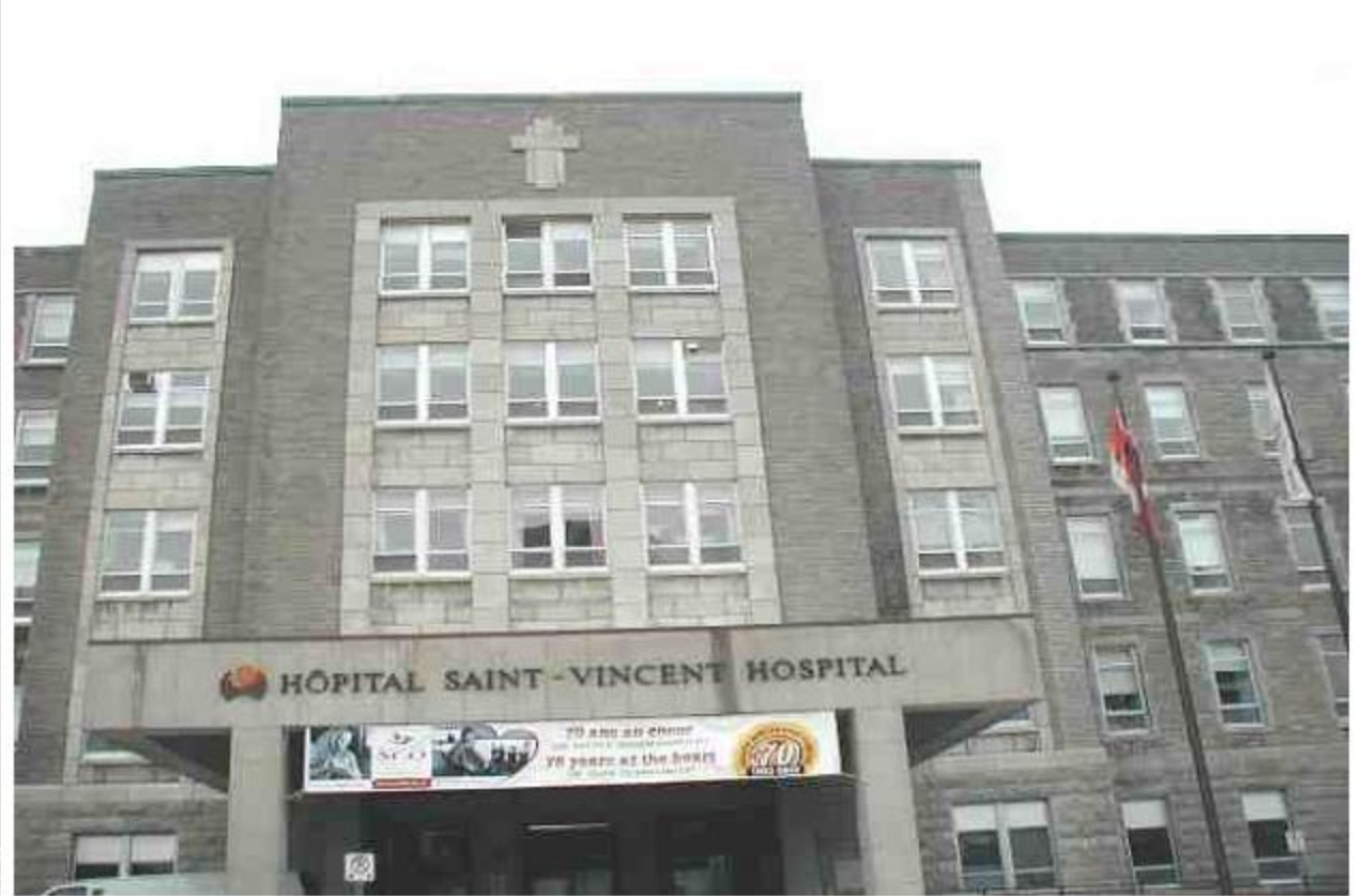
Figure 1, Front View of Wing-B (Partial)
