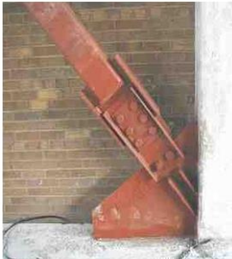
Friction damper in single diagonal bracing
